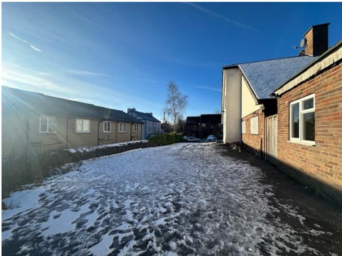
Image 4: view of Spring Court Mews from existing hardstanding area to south of plot
